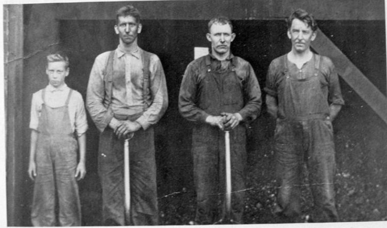
#6 Powerhouse. Right to left: Bailey Stephens, David Stutzman, Wilbur Stutzman, _____ Kempfer. Courtesy of Dorothy (Stutzman) Stephens.
